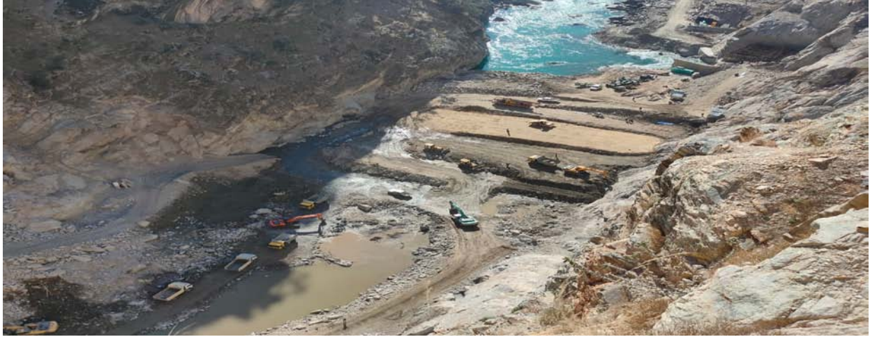
COFFER DAM & DAM EXCAVATION
