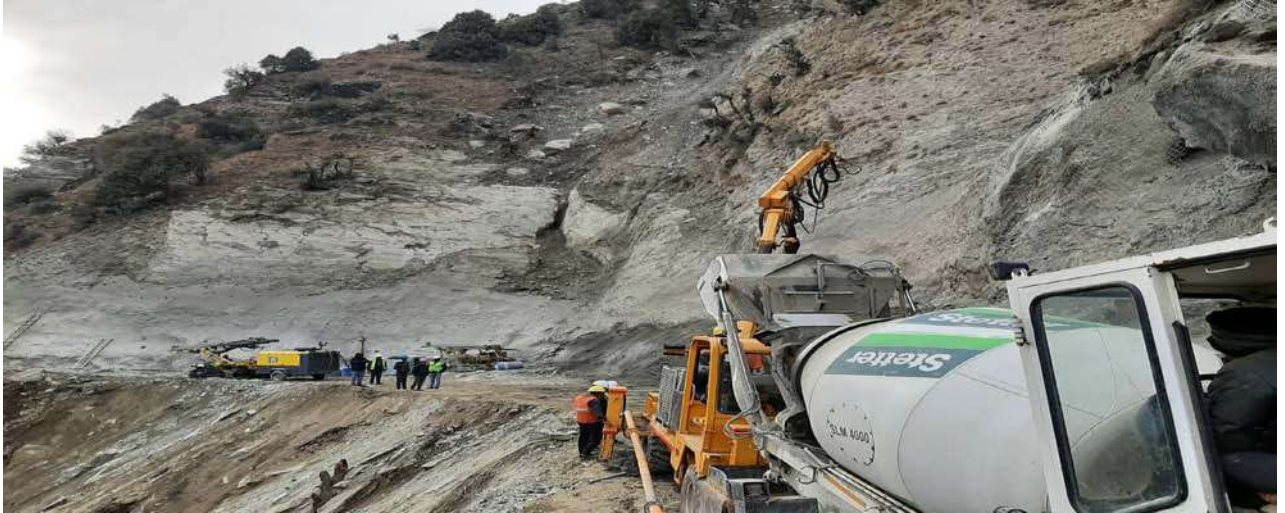
TBM Adit Portal Area
