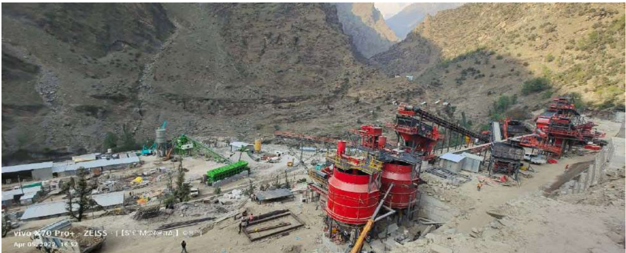
Erection of 600 TPH Crusher Plant
