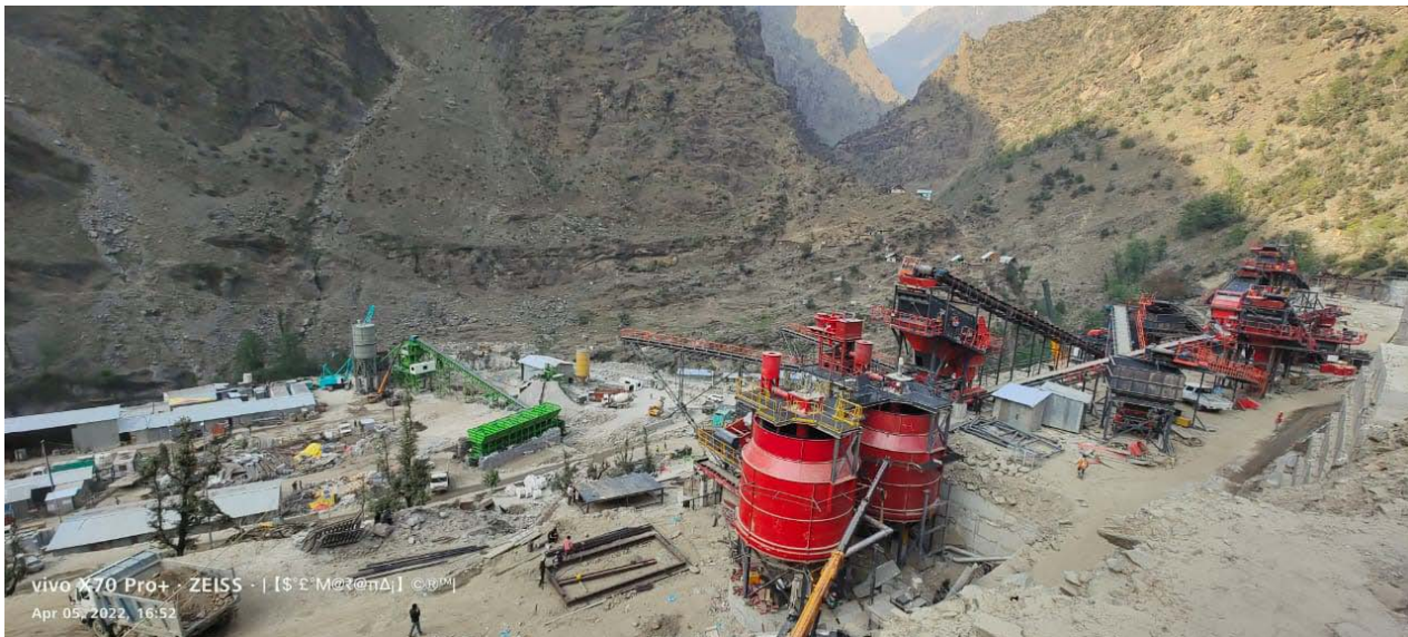
Erection of 600 TPH Crusher Plant
