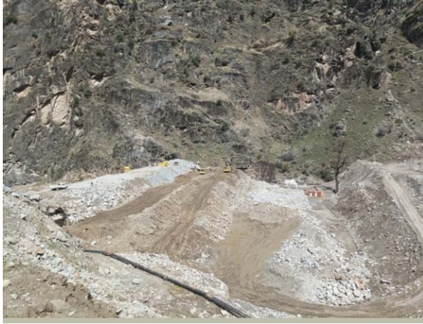
U/s Cofferdam filling
