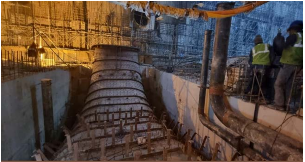
Erection of Draft Tube # 3
