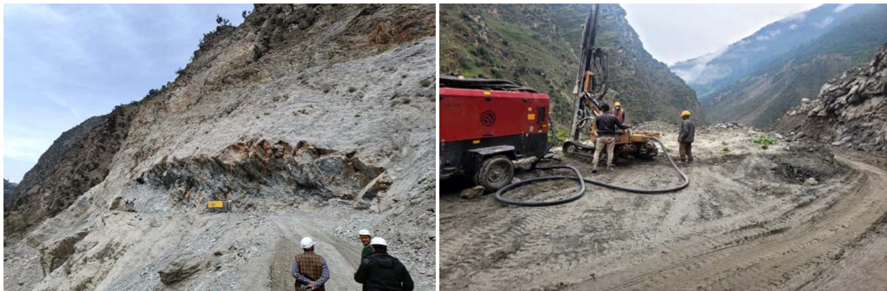
Construction of TRT Adit Road
