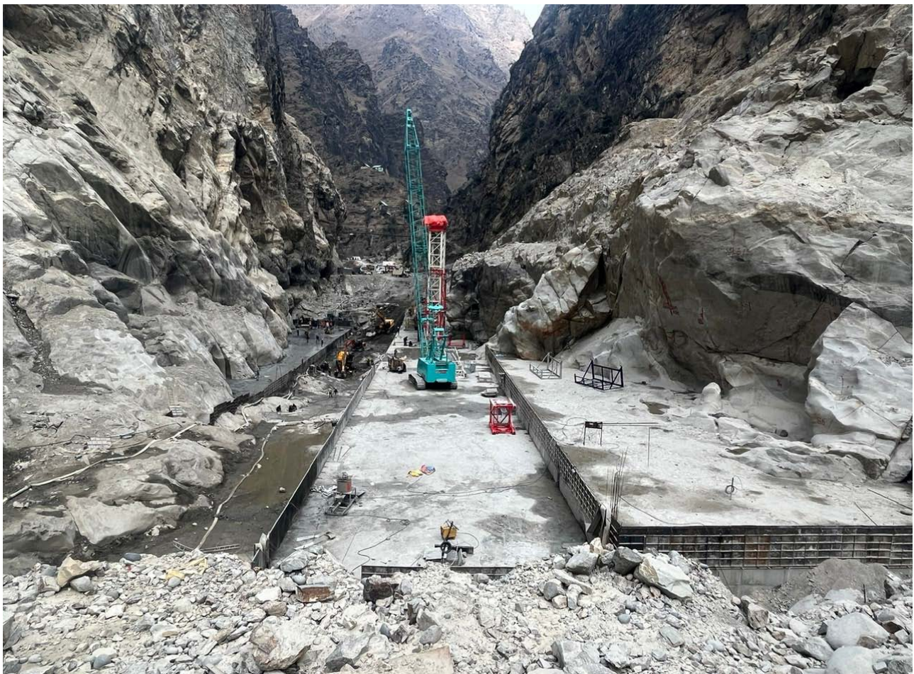
Dam upstream view
