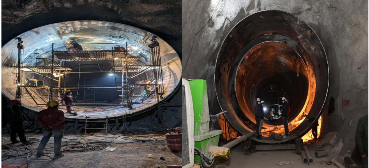
Upper Horizontal Pressure Shaft Steel Liner PS2
