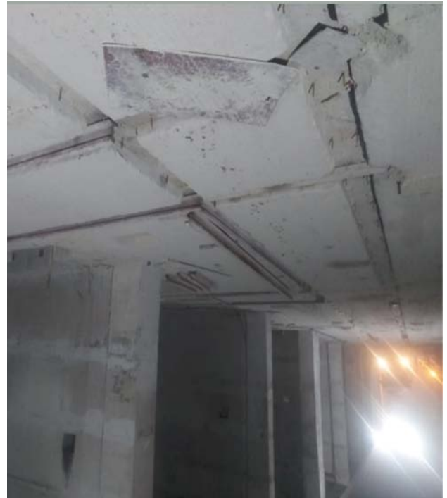
Installation of GT Rail line
