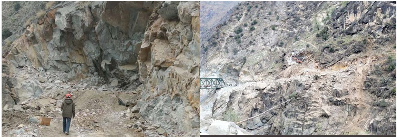
DAM Axis Road on Right bank
