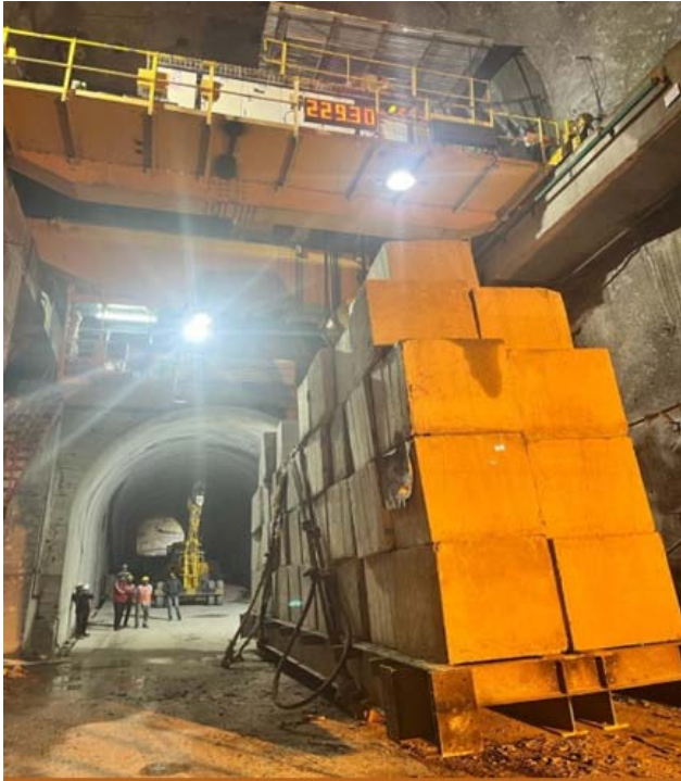
Load test of MIV EoT crane
