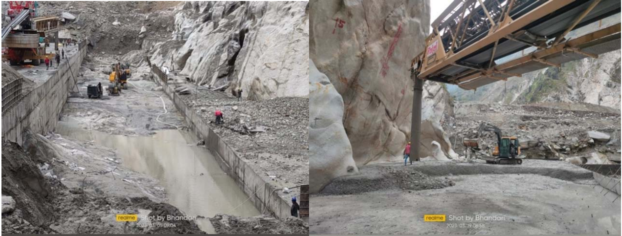
River Bed Excavation Concrete pouring in S5 block
