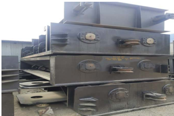
Diversion Tunnel Gates Received at Site
