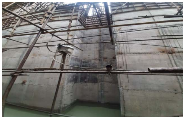
Erection of 1st Stage Embedded parts at Diversion Tunnel Gate Shaft
