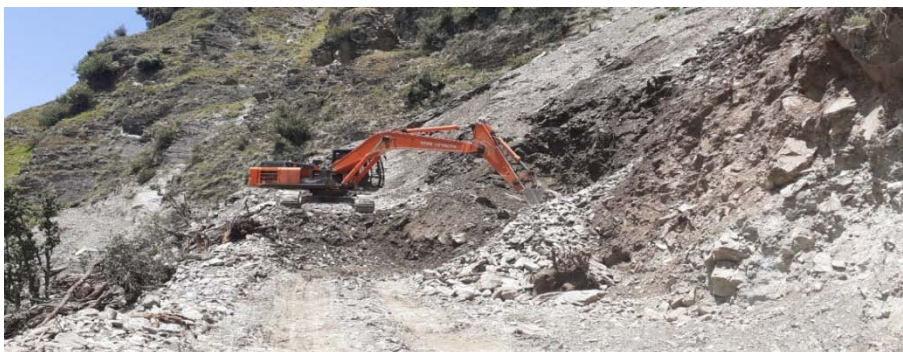
Excavation for development of TBM Launching Platform for HRT Excavation
